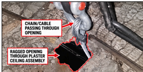
1 PLENUM-SIDE VIEW OF RAGGED OPENING THROUGH HISTORIC PLASTER CEILING ASSEMBLY.
