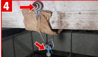
THREADED CONCRETE-BEAM THROUGH-BOLTS AND WIRE-ROPE RIGGING CONNECTIONS.
