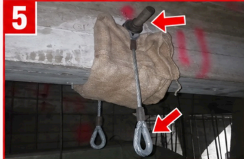
THREADED CONCRETE-BEAM THROUGH-BOLTS AND WIRE-ROPE RIGGING CONNECTIONS.
